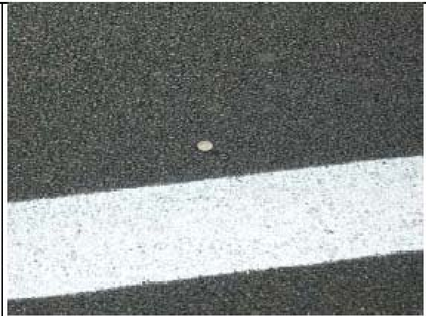
Rubberized Asphalt Concrete (RAC-O) Post-Construction Pavement, January 2008
