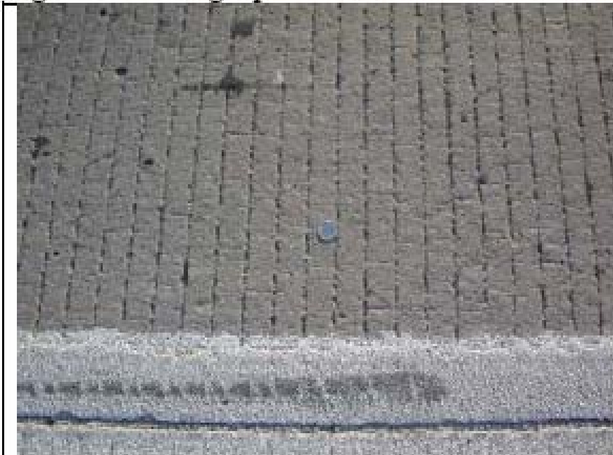
Uniformly Transverse Tined PCC (PCC) Pre-Construction Pavement, November 2006
